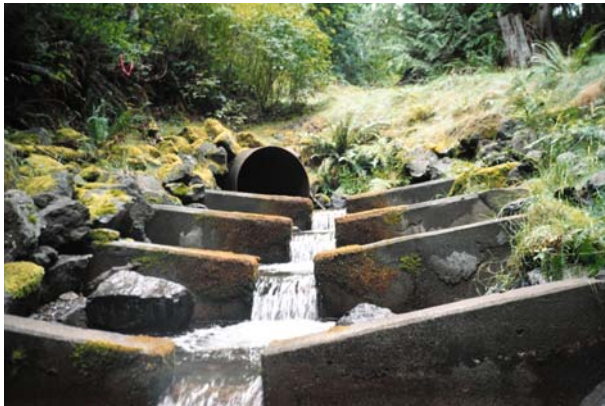
Culvert on Dickinson Creek, Kitsap Peninsula.
