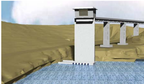
Howard Hanson Dam before construction of the fish facility.
